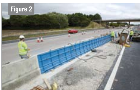
Fixed formwork for bifurcation
