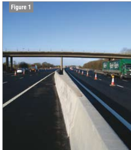
Asymmetric bifurcation at bridge pier
